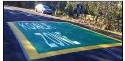
*Pavement treatments reiterate the commencement of the koala road. The design is consistent with treatments used in other locations for wildlife zones.*
